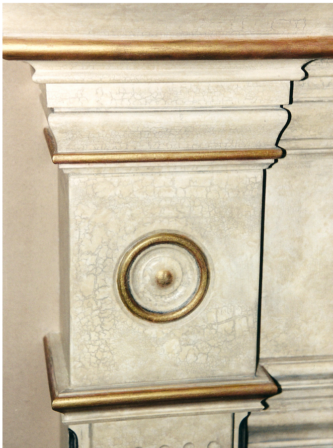
Metal Leafed Molding Detail
